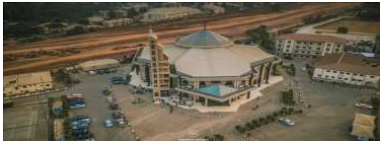
Fig 1: Landscape facade of Our Lady Queen of Nigeria cathedral (Source: Wikipedia, 2025)
