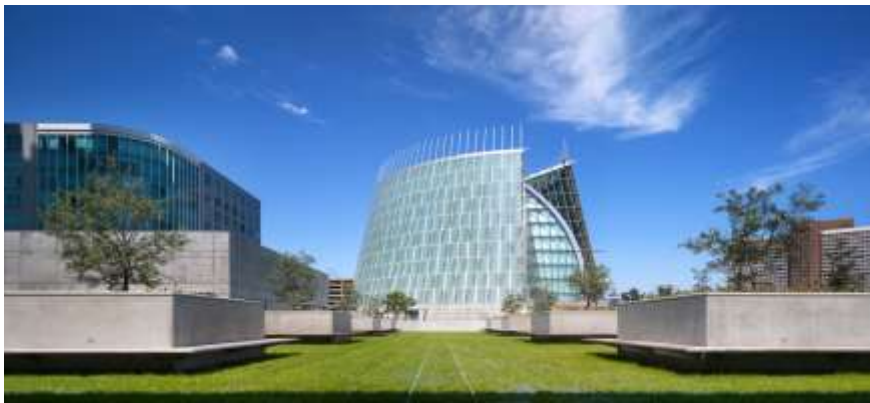
Fig 5: Landscape facade of The Christ cathedral (Source: Archdaily)
